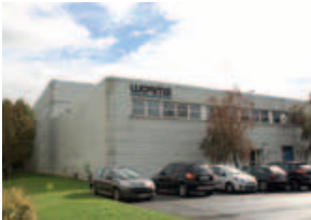
IMER France - WORMS Entreprises Power Generators Paris, France
